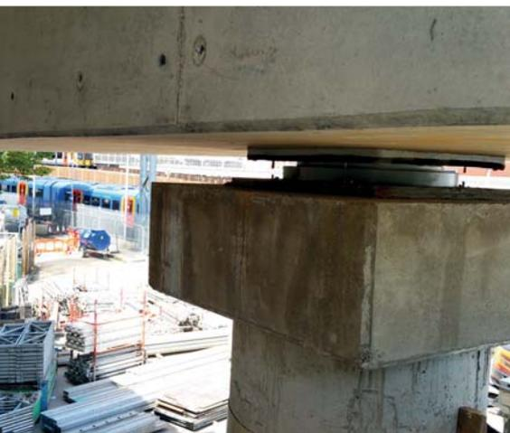
Structural bearings supporting transfer beams.
