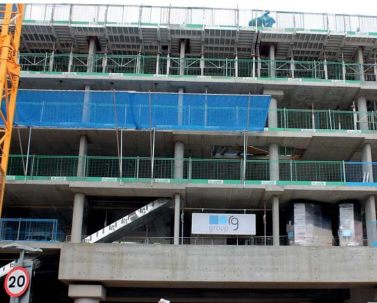
RC frame and short-spanning grids above transfer beams.
