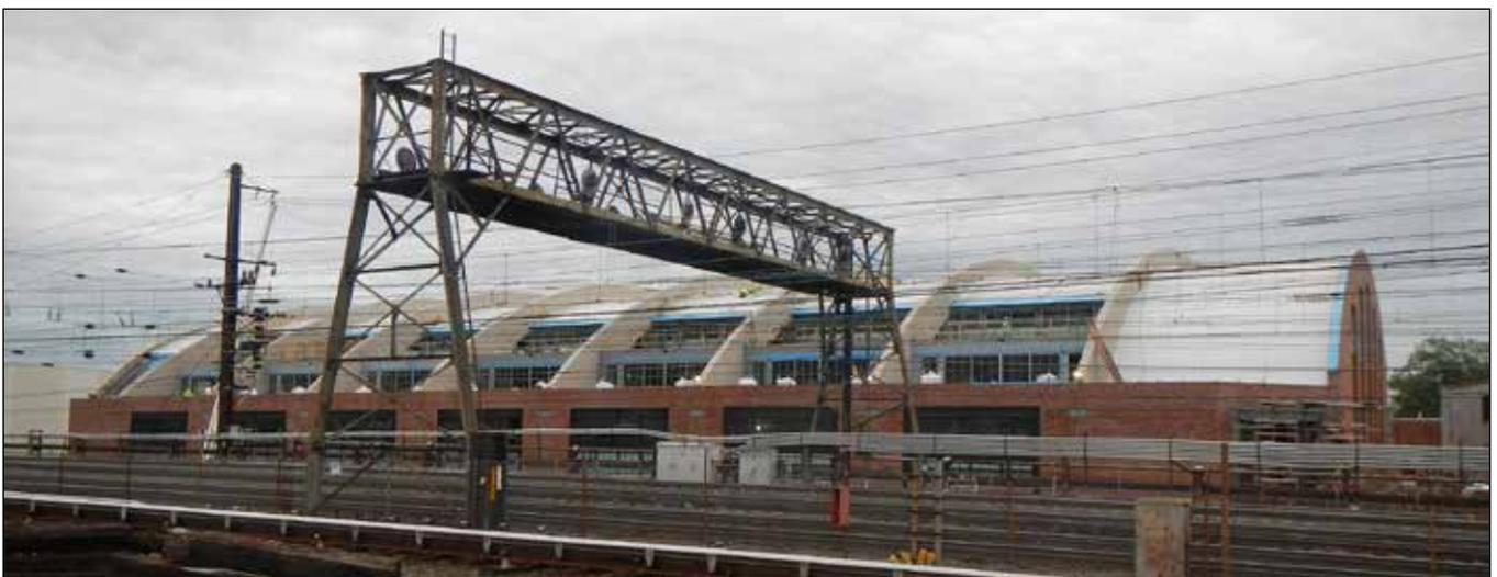
formed of thin sprayed concrete panels supported by external concrete arches that sit on concrete columns.
