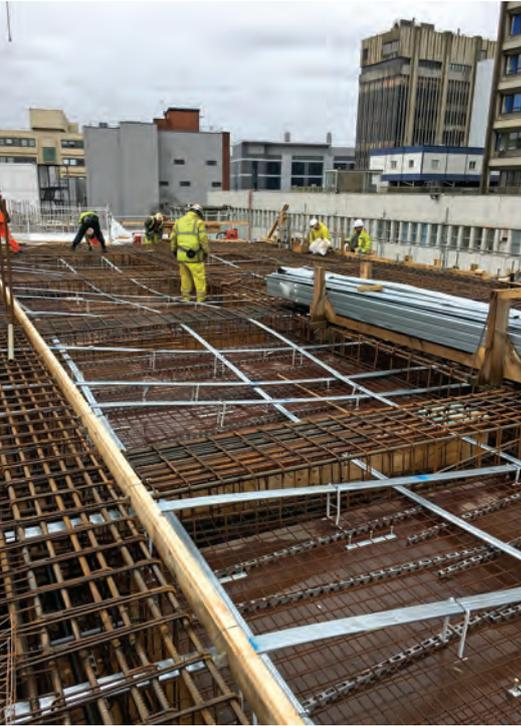
PT tendons in the MRI area where deep orthogonal beams are located.
