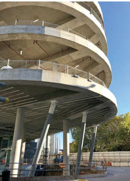
The prow of the building showing the cantilever slab, inclined columns and the orthogonal beams.
